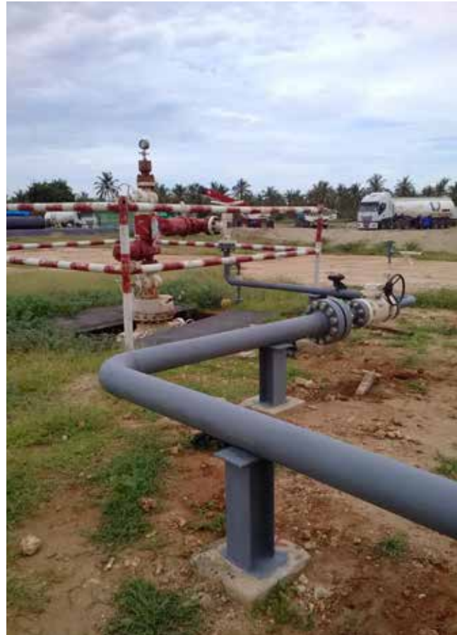
Temporary connection to well head at Mnazi Bay Natural Gas Field.
