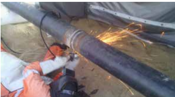
Welding of Natural Gas Pipes and Fittings
