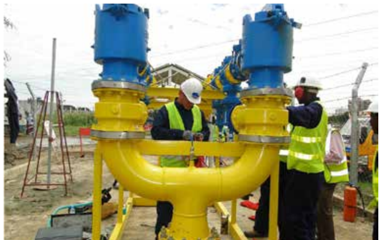
Setting Outlet Pipeline Pressure at Pressure Reducing Station
