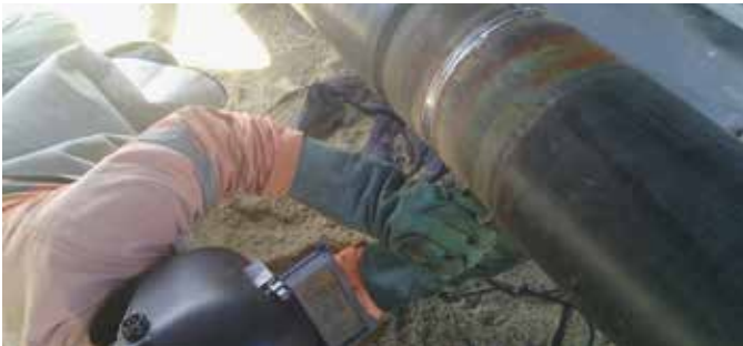
Pipe welding work for Replacement of 8 Inches Submarine Pipeline at Mtoni, Zanzibar for transportation of Jet-A1 fuel for PUMA Energy Tanzania Ltd
