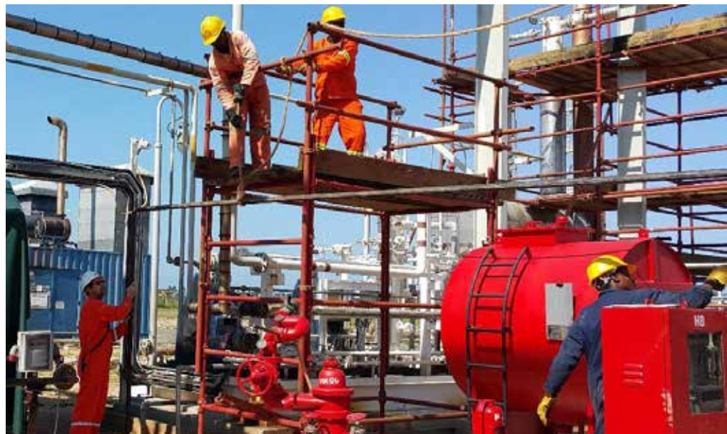
Handling & lifting of Rich Jump-Over Spool for installation
