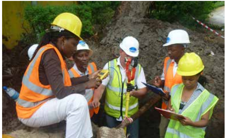
Natural Gas Pipeline Integrity Tests During construction of a 7.7Km natural Gas Pipeline from Ubungo to Mikocheni for TPDC
