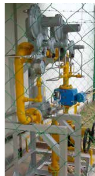
Improvement of Pressure Reducing Station at TPDC Village, Mikocheni
