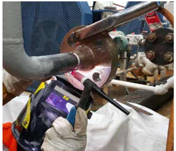
Welder Damian Samson (W8) performing tack welding onto Joint No. FW-L1 (tie-in golden weld)
