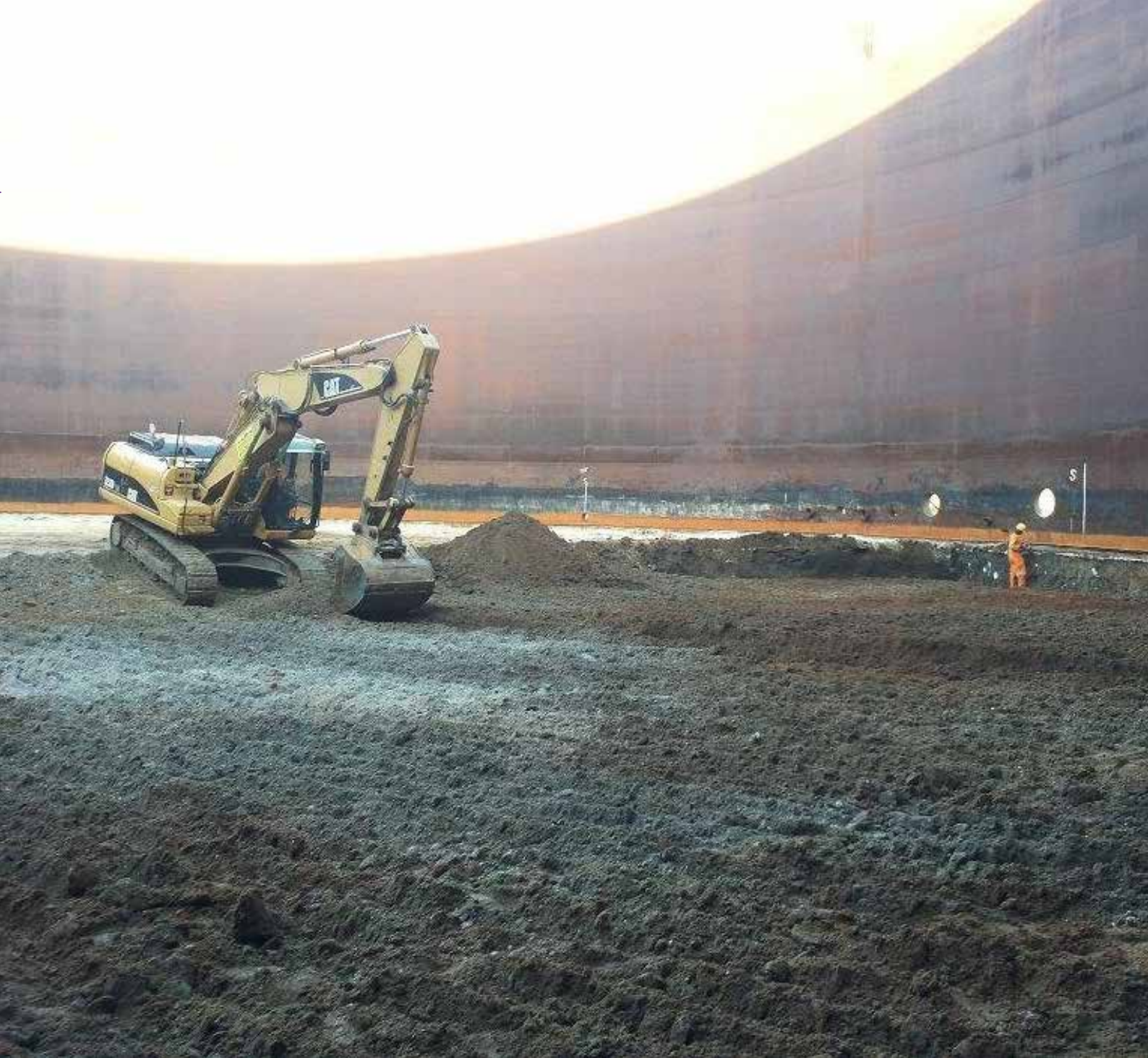
Civil Works on Rehabilitation of 36 million litres Fuel Storage Tank for Tanzania International Petroleum Reserve (TIPER)
