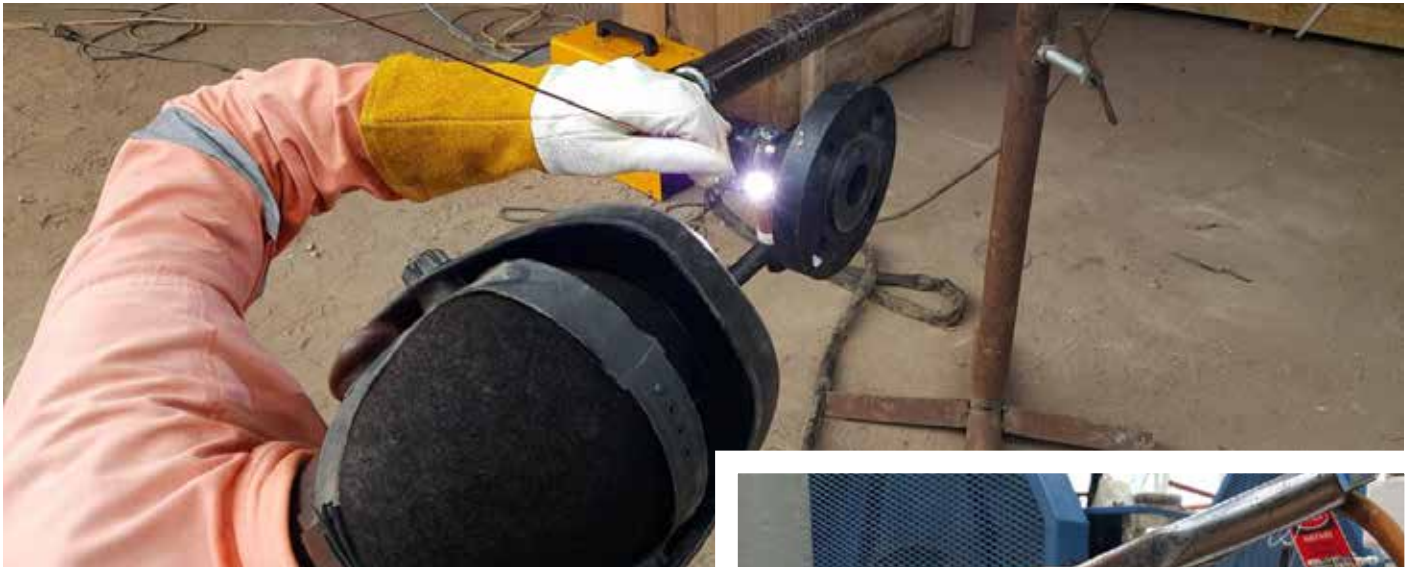
Welder Ismail Mbinga (W10) welding Weld Neck Flange onto Rich Spool Elbow Section
