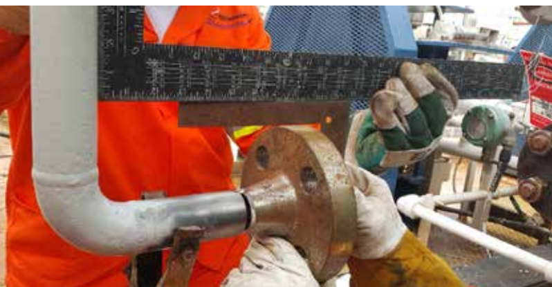
Dimensional checking in progress during fitting of new 1,500lb weld neck flange onto existing Lean Piping by Fitter Edwin Mtaki
