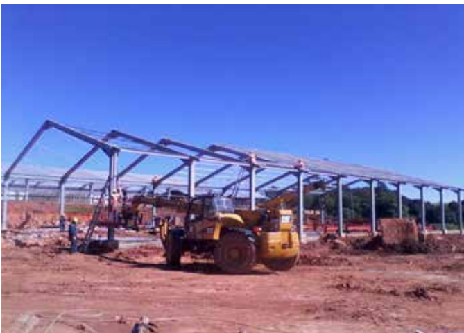
Ongoing Construction of Kibwele Tea Factory at Mufindi, Tanzania for Unilever Tea Tanzania Ltd
