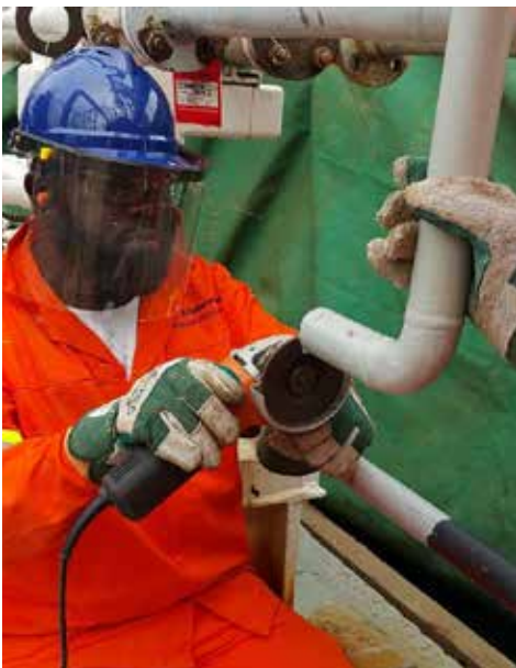
Grinding preparation of field weld (golden weld) Joint No.: FW-L1
