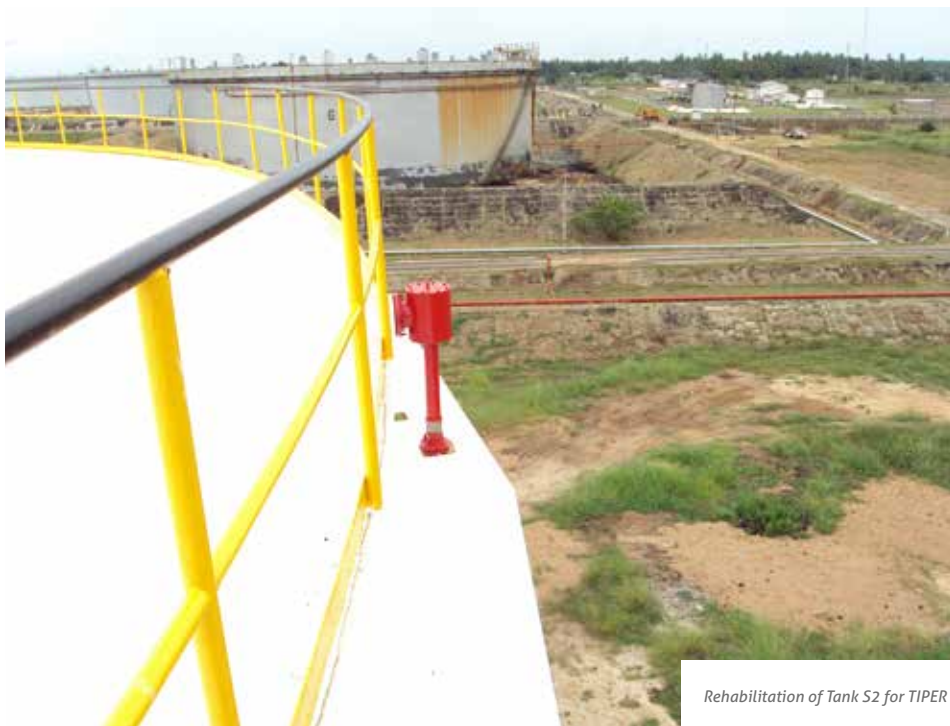
Construction & Rehabilitation of Fuel Storage Tanks
